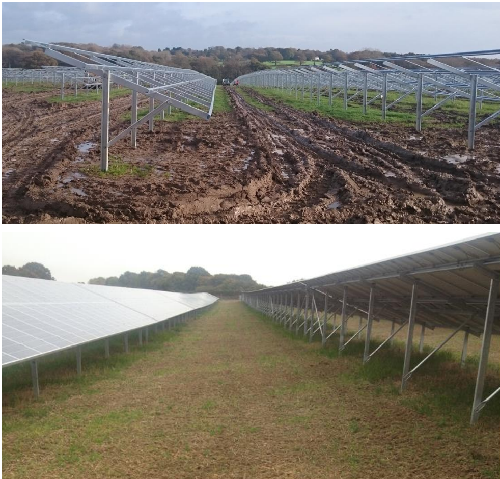
Inserts 26 and 27: Inter-row Ground Restoration
